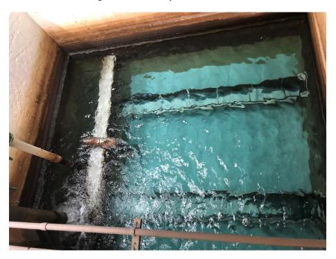
Figure 2-15: Gravity Media Filter Cell
