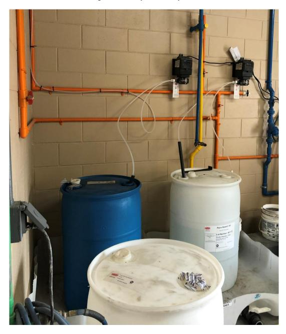
Figure 2-22: Polymer Feed System
