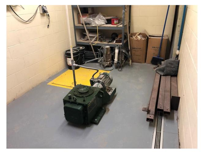
Figure 2-14: Existing Recarbonation Basin Mixer Drive
