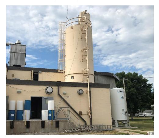
Figure 2-18: Hydrated Lime Silo
