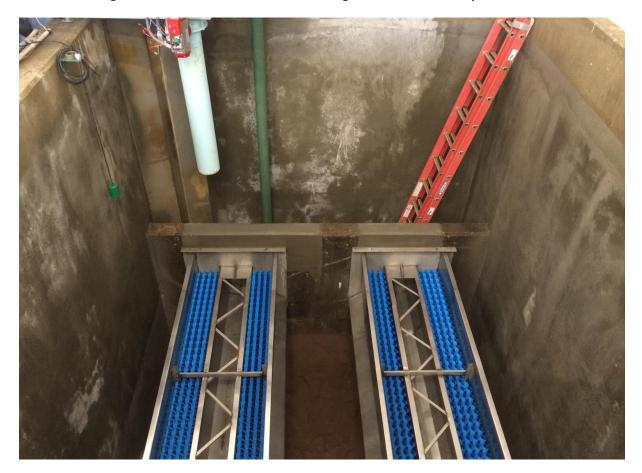
In order to improve the backwash system, a means to provide adequate backwash volume is needed. As previously shown, the current method of backwashing provides inadequate volumes of water needed to thoroughly clean the filters. This alternative includes the installation of either a new backwash pump or piping and valving required to use distribution system water for backwashes. The exact method used would be determined in design.
