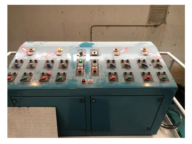
Figure 2-23: Current Filter Control Panel
